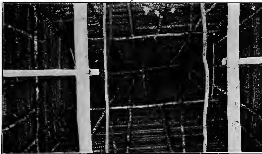
CONSTRUCTION OF ROOF OF A NATIVE HOUSE
